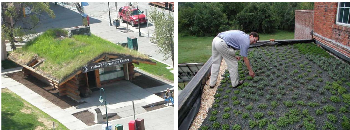
Fig. 10: A turf covered green roof in Alaska is very attractive (left). A similar green roof in North Carolina would require irrigation. A succulent (sedum) vegetated green roof is shown in Kinston (right)
