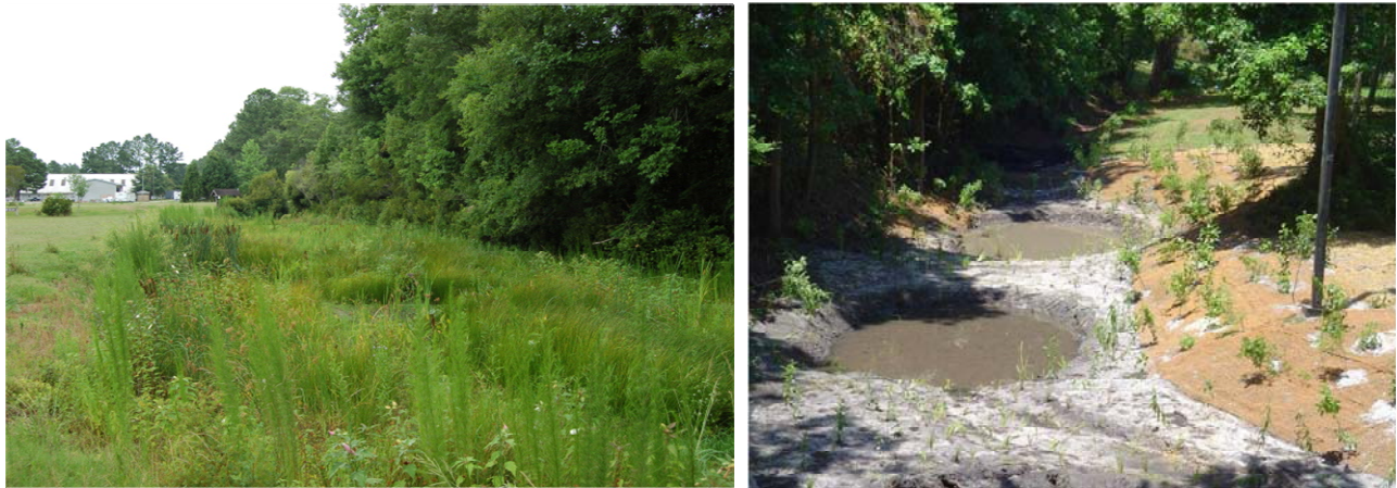
Fig. 2: Two infiltrating wetlands located in North Carolina (a) River Bend and (b) Wilmington. In (b) the inundated deep pool is in contrast to the remaining portion of the wetland which is not saturated at the surface
