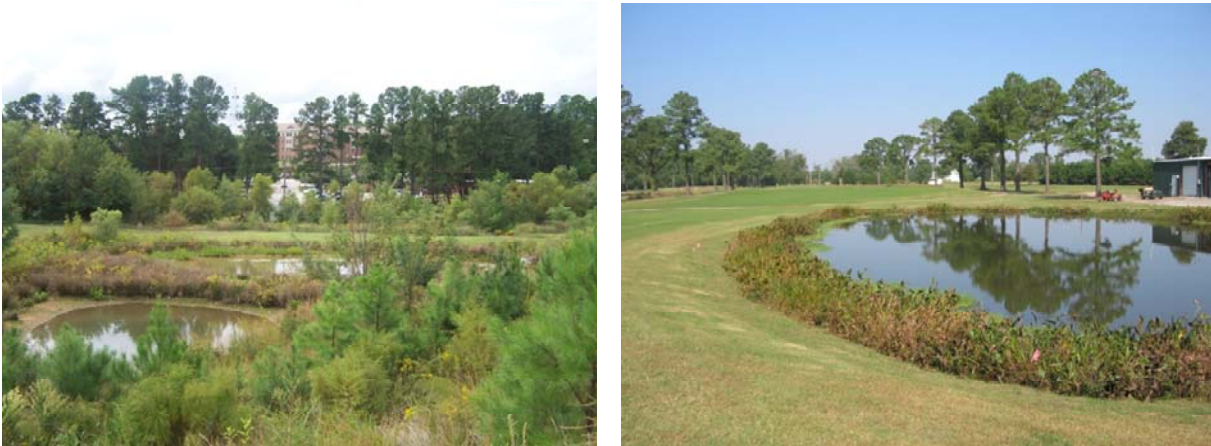
Fig. 1: Wet Ponds with forebays (left) and aquatic shelves (left and right)
