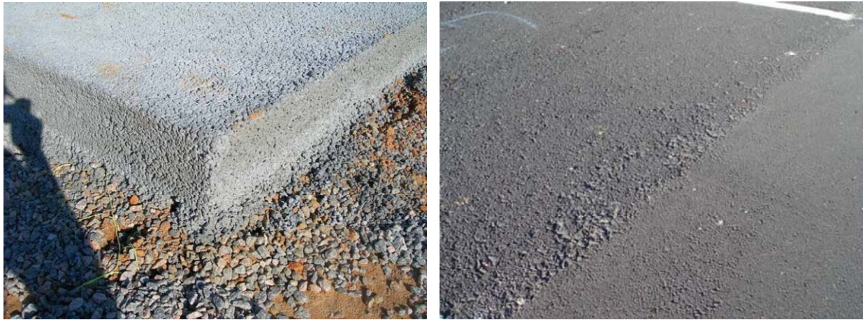
Fig. 9: Pervious concrete used in Nashville, NC, (left) and pervious asphalt found in Raleigh, NC, (right) are two types of permeable pavement
