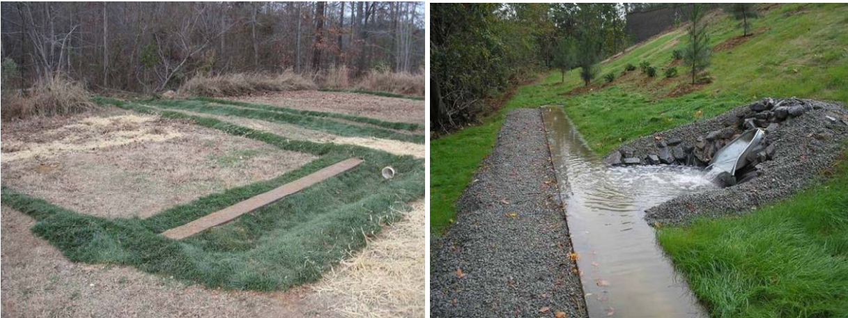
Fig. 6: A pair of level spreaders in Apex, NC. Each is made of structurally durable and level material: concrete (left) and metal (right)
