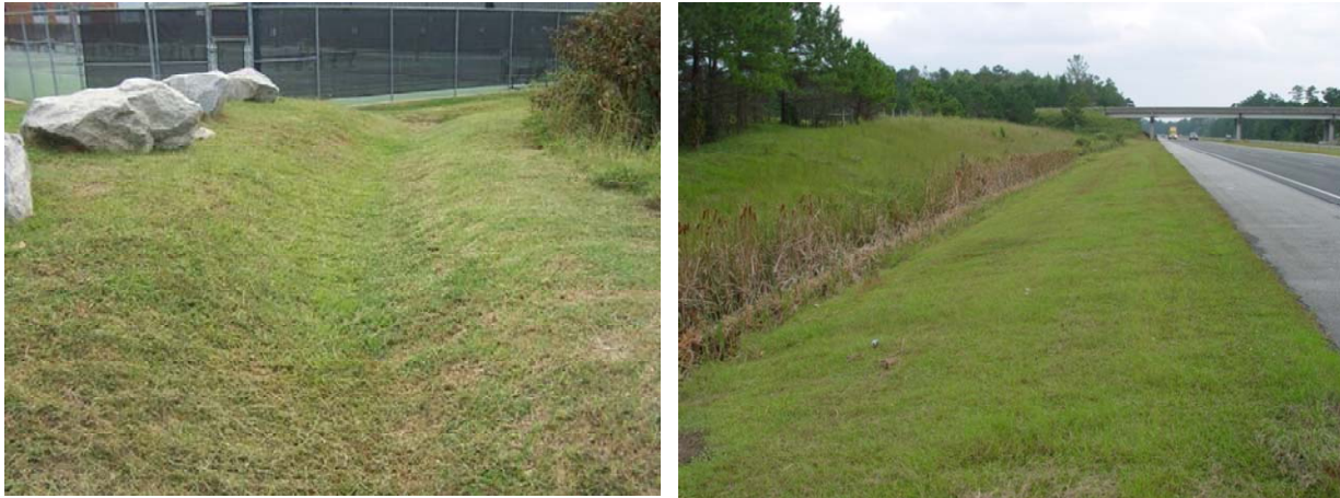
Fig. 7: Two swales, one dry (in Raleigh, NC) and one wet (along I-40 in eastern NC) are used to convey water
