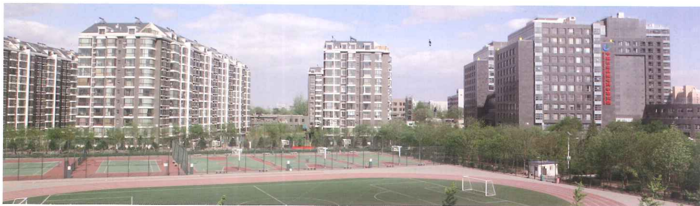
Bird's-eye View of the Campus of CAAMS
